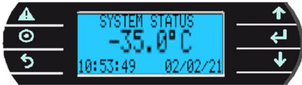
Panel front view
